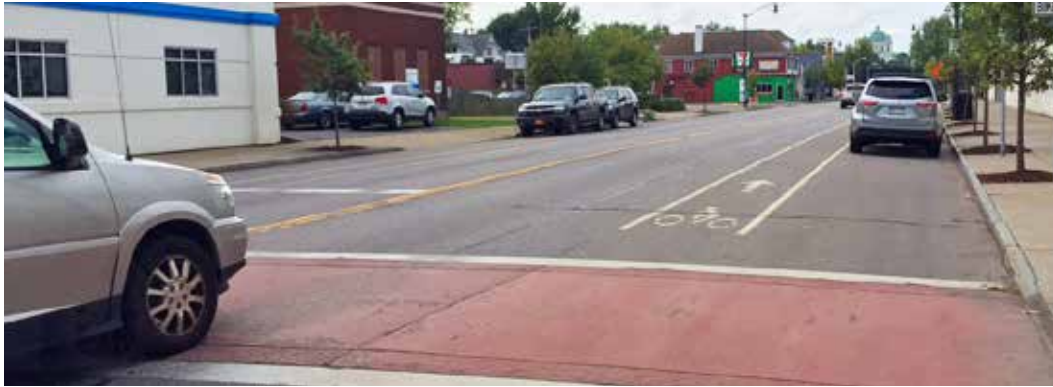
Image 32: Complete Street Infrastructure at South Park Avenue
