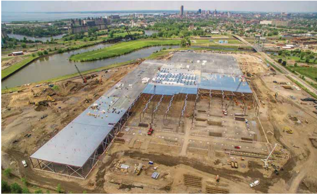
Image 20: Buffalo High-Tech Manufacturing Innovation Hub at RiverBend under construction
