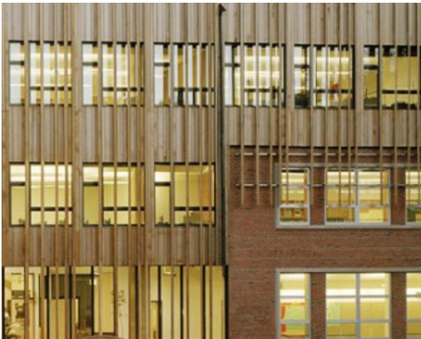
Wood and masonry siding used together with glazing
