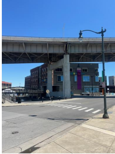
View North From Marine/Commercial
