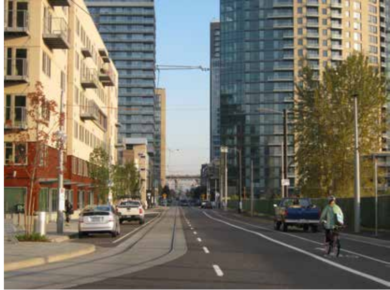
Narrow lane widths and curb extensions can help to support additional street facilities such as bike lanes or on street parking
