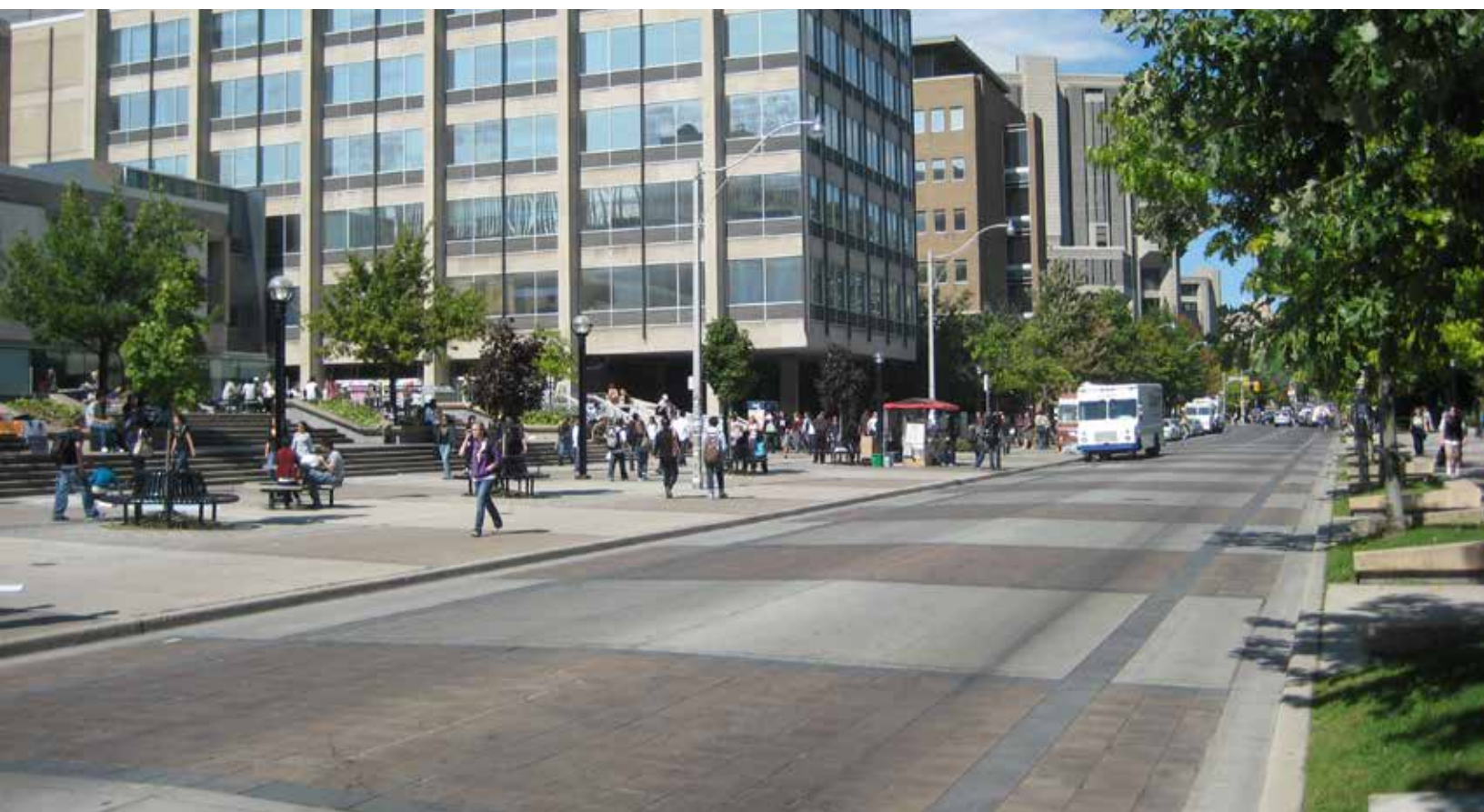
Speed humps, traffic tables and changes in materiality can heighten driver awareness in areas with high levels of pedestrian activity
