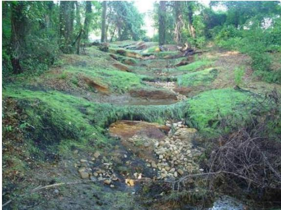
Figure 44. Regenerative Stormwater Conveyance outfall treatment, *Photo Biohabitats*
