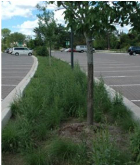
Figure 27. Bioswales between parking bays.
