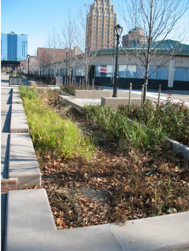
Figure 37. Biofilter planter in Buffalo. *Source: Buffalo Niagara Riverkeeper*
