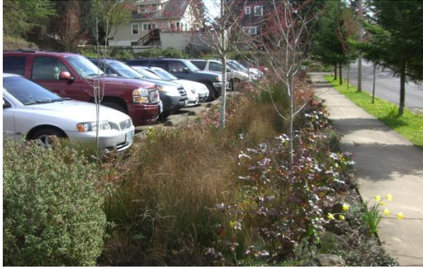
Figure 26. Bioswales along the edge of a parking lot. *Photo by Biohabitats*
