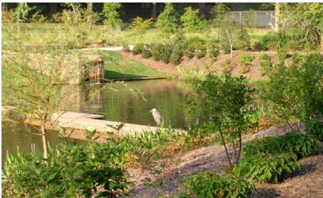
Figure 41. A stormwater wetland with a more formal edge. *Copyright Biohabitats*
