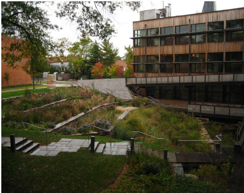
Figure 47. A photo of the completed alternative wastewater treatment system at the Sidwell Friends School. *Copyright NSI*
