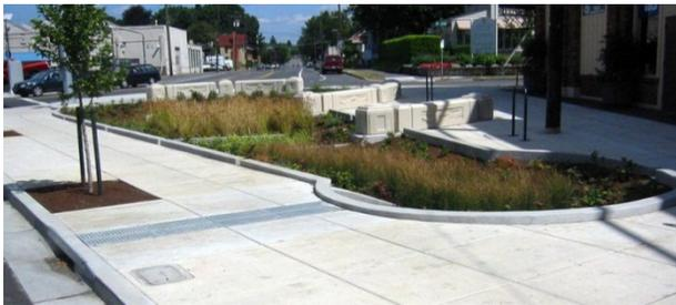
Figure 38. Biofilter planter. *Source: Allegra Bukojemsky*
